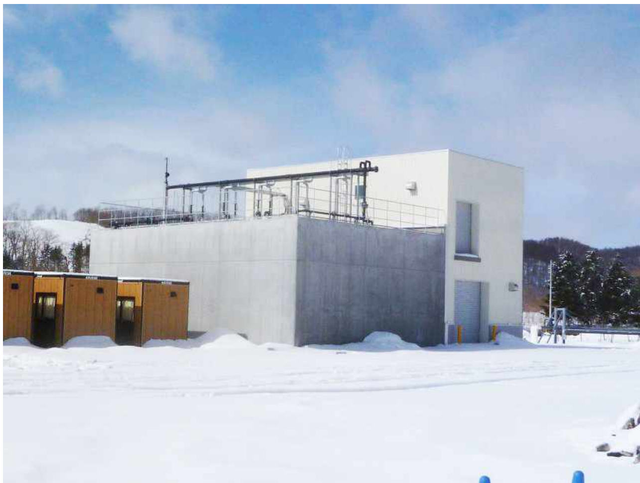
New membrane tank
