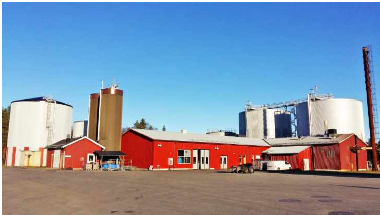
Biomar® wastewater treatment plant with 2 Biomar AWR-reactors (right) and a Biomar OSB-reactor (left)
